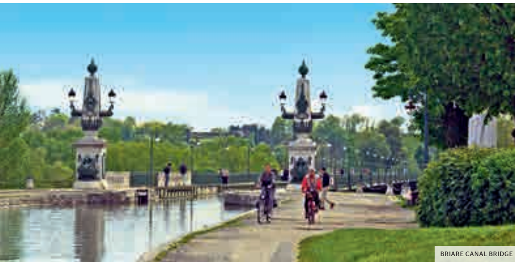
BRIARE CANAL BRIDGE
